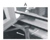
Adjustable hinge track (optional) allows user to compensate for sash sag. Top and bottom hinges are adjustable with use of available stud wrench.
